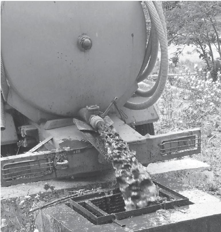
Photo 6.1 Direct discharge to an Imhoff tank: an unsatisfactory arrangement resulting in spillage
