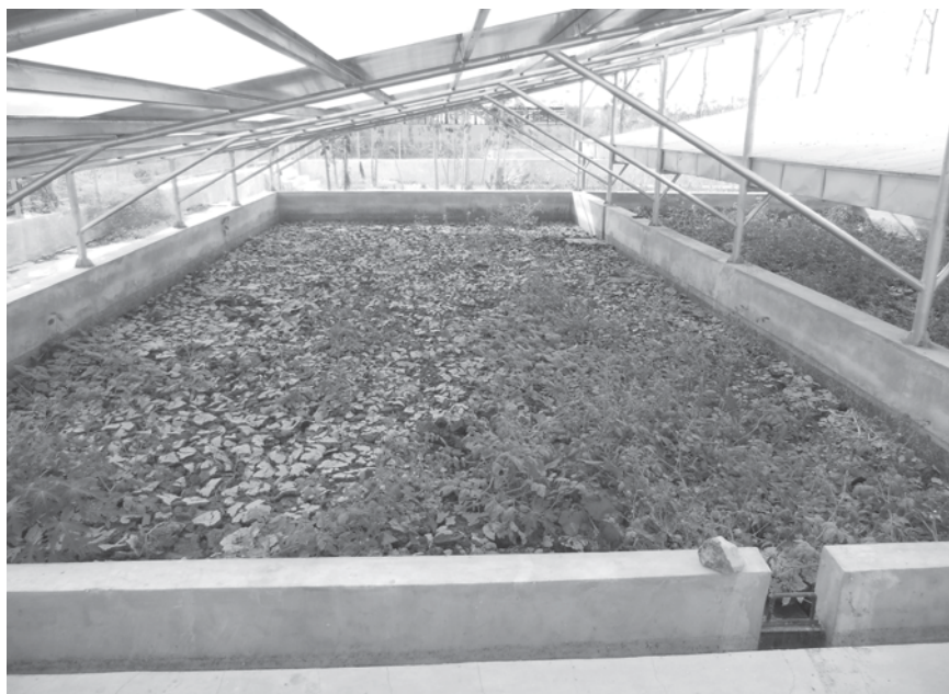
Photo 9.2 Drying bed cover arrangement, Jombang, Indonesia
