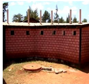
Figure 2: Large-scale bio-latrine system showing the Biogas and toilet structures. Photo credit: Practical Action Kenya.
