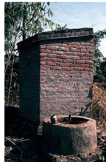
Figure 1: Household Bio-latrine showing toilet attached to a bio-digester Photo credit: Practical Action.
