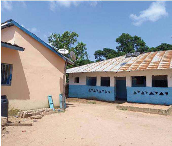
Fig. 3.3 The same school is also equipped with Baobab+ solar panels to cope with the mini-grid unreliability (Field Study in Southern Senegal, 2021)
