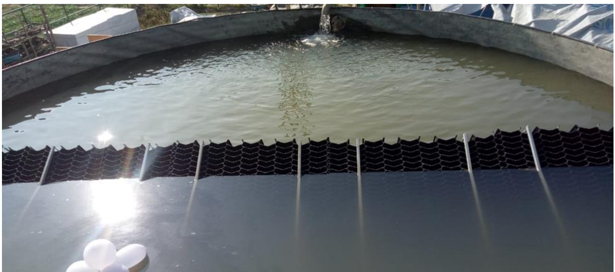
Set-up for T70 tank in Bangladesh. The honeycomb shaped lamella "boxes" comprise lightweight polypropylene single channel tube profiles with "tongue and groove" joints which are then heat welding. This enables them to be supplied as kits and erected on site.
