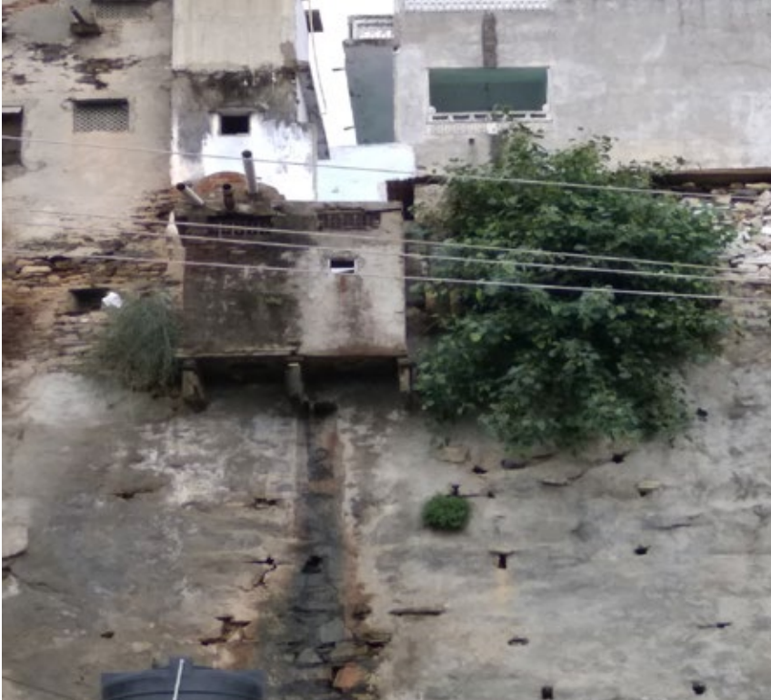
Fig. 5: Toilets Built Hanging Out and Releasing Faeces on to the Ground below
