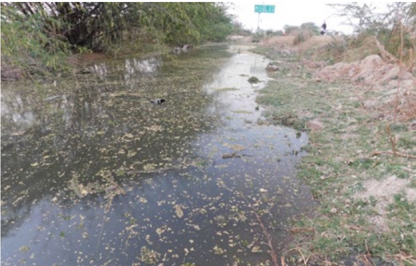
Fig. 8: Untreated Wastewater flowing along the Highway in Kekri Town
