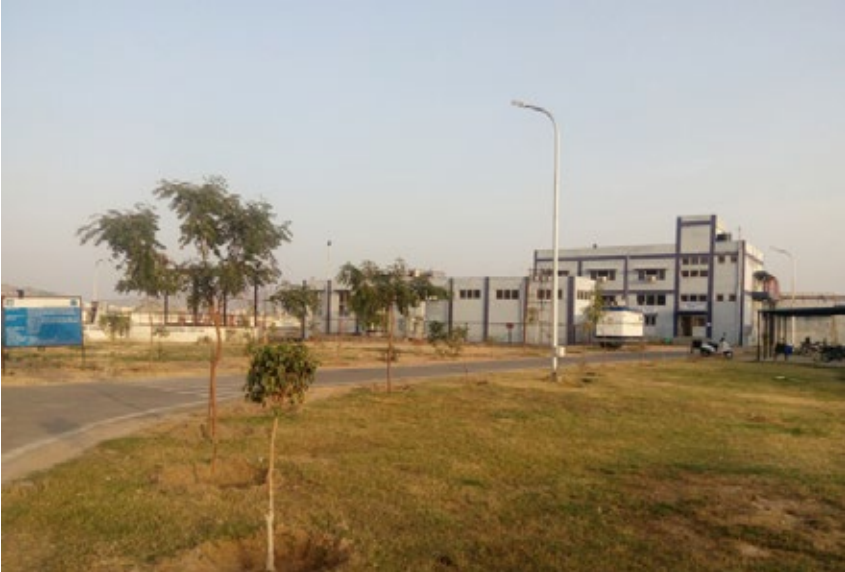
Fig. 9 : 13 MLD Sewage Treatment Plant at Anasagar Ajmer
