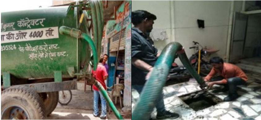
Fig. 6: A Private Septic Tank Cleaning Machine in operation
