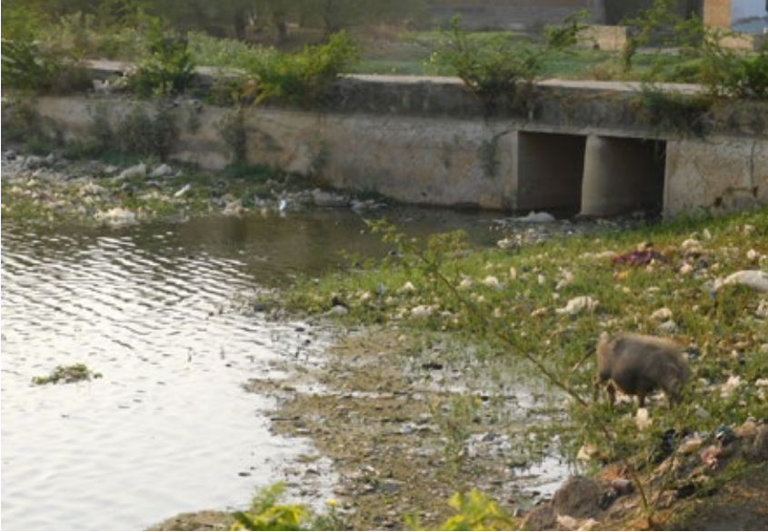
Fig. 7: Drain flowing into the Bada Talab Pond in Kekri
