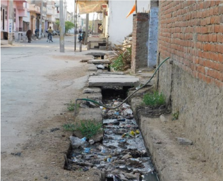
Fig. 6. Open drain in Kekri Town
