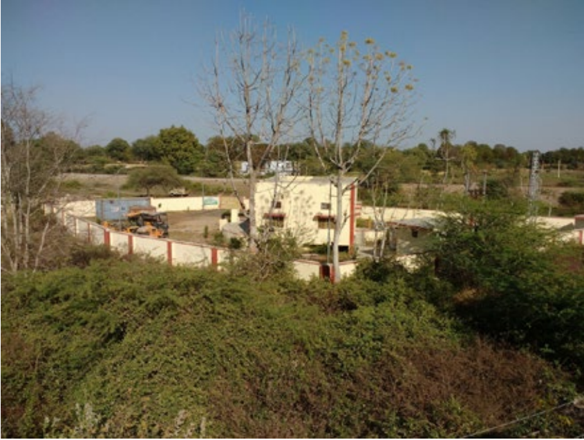
Fig. 7: Sewage Pumping Station at Taledi Nala in Rajsamand
