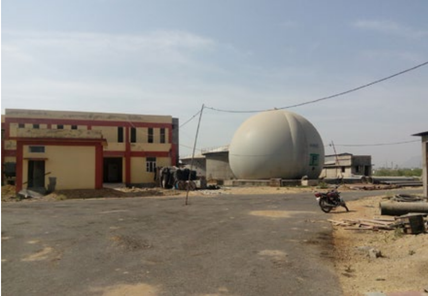
Fig. 10 : 40 MLD Sewage Treatment Plant at Khanpura Ajmer
