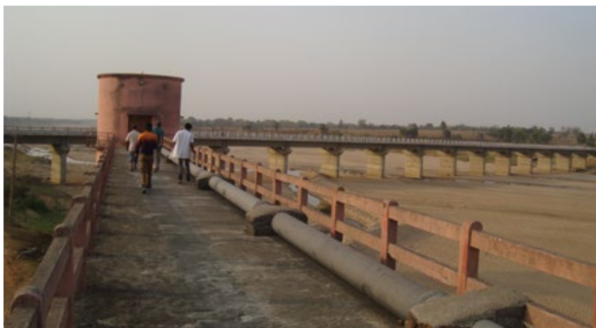
Ajay River Pump House
