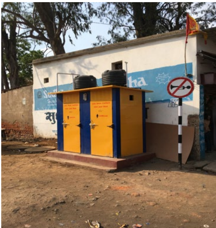
Community Toilets built as part of SBM
