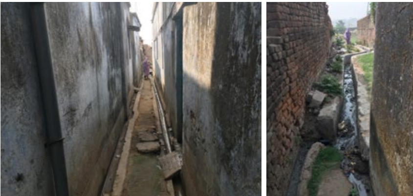
Drains in Mihijam
