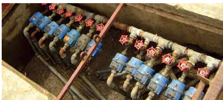
Meter chamber on Line 1
