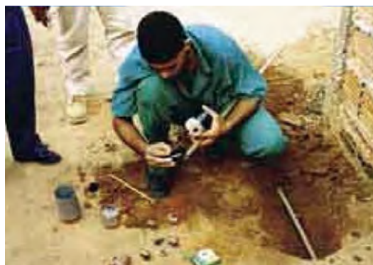
Installation of micro-meter in household connection, Parauapebas
