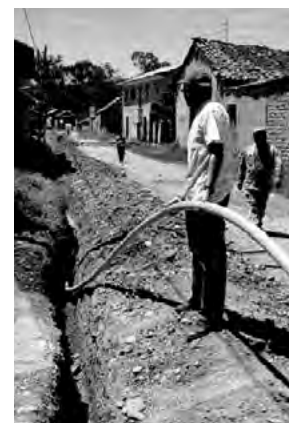
Laying of a pipeline
