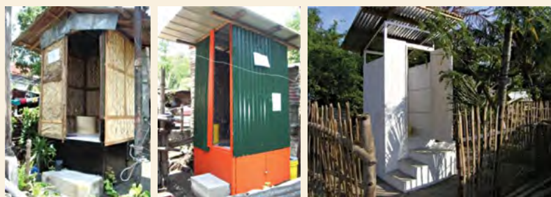
Construction of UDDTs in various materials
