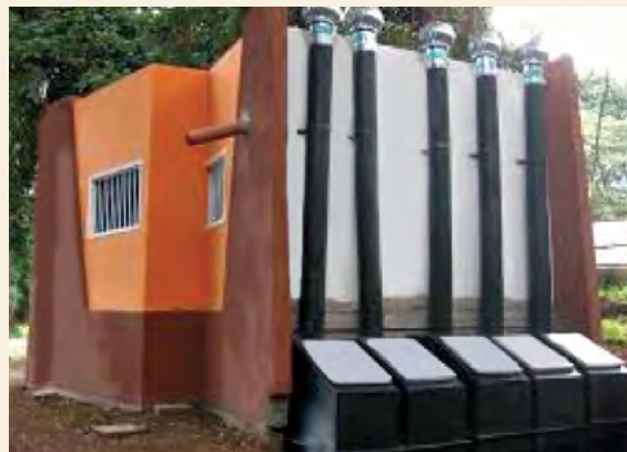
Ikotoilet Urine Collection System, City Park, Nairobi
