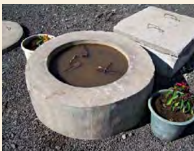
Area of top manhole, above the Biogas Dome
