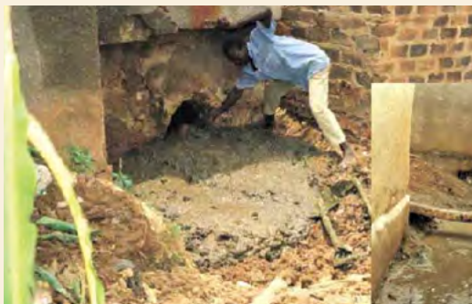
Manual pit emptying: unsafe and unhygienic
