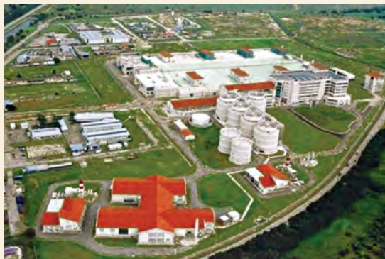
Changi Water Reclamation Plant
