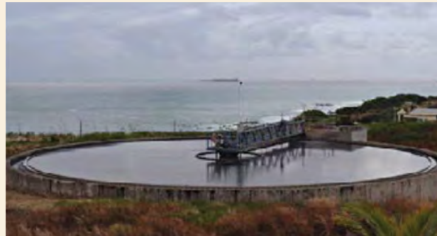
Wastewater Treatment Plant
