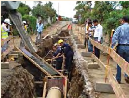
Construction of Sewerage System
