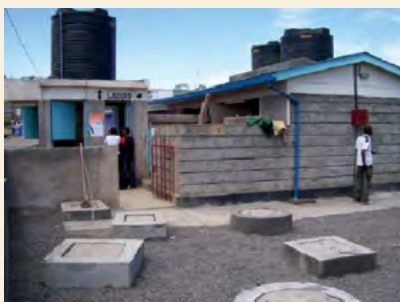
New Public Sanitation Facility
