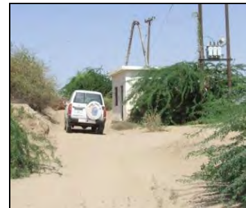
Free access to water extracting and pumping facility
