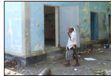
Dirty and crowded floors & walkways in chlorination facility obstructing the work
