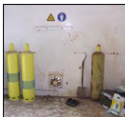
Poorly maintained chlorination facility; while the safety signs are wall mounted (good practice)
