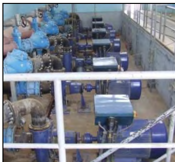
Powerful machines with high speed rotating parts un-covered
