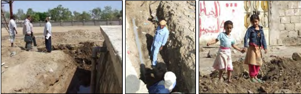
Excavation without installing barriers or supports (shoring) is wrong; workers or third party may fall into excavations and/or excavation sides may collapse and bury employees
