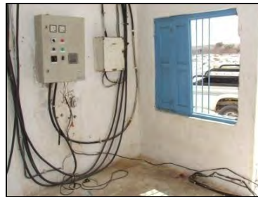
Wiring in a remote and un-manned site, some are exposed
