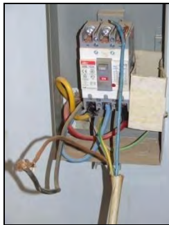
Exposed electrical wire may cause shock to employees if they touch it
