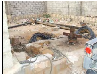
Chaos on floor & walkways of water extracting site may cause fall and harm
