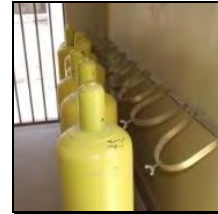
1- loose cylinders. (deficiency) 2- Vertically fitted to the wall chlorine cylinders (good practice)
