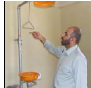
Safety shower found disconnected of water resource by a tap, it will not help during emergencies
