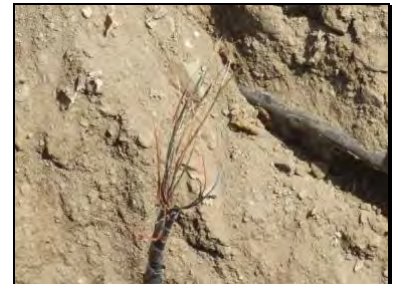
Not using cable locator before excavating resulted in cutting the cables
