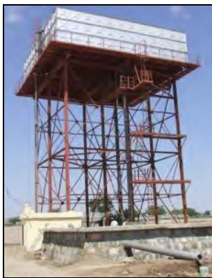
Uncontrolled access to a tower reservoir
