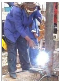
Welding without protection against fumes
