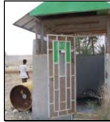
Out-of-use chlorine room left without control or maintenance for a long time
