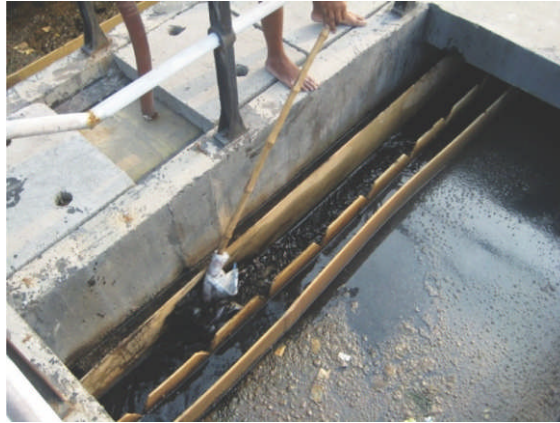
Figure 4.22 Cleaning of effluent gutters
