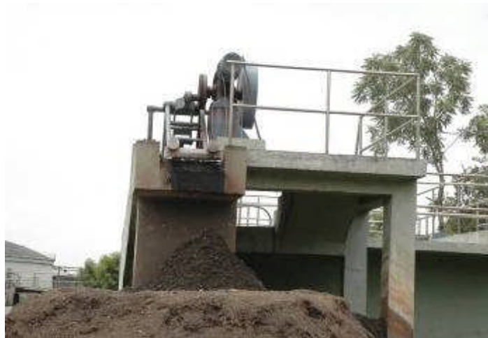
Figure 3.13 Typical grit chamber
