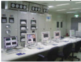
Figure A1.1-3 Central Control Room
