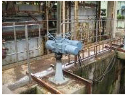
Figure 3.7 Electric motor driven gear actuator
