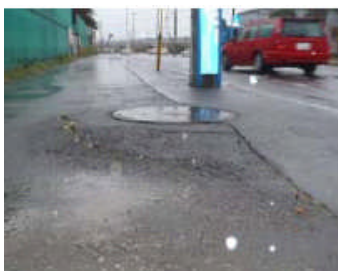
Figure 2.39 Not coinciding with height of road surface
