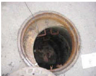
Figure 2.38 Offset of manhole block
