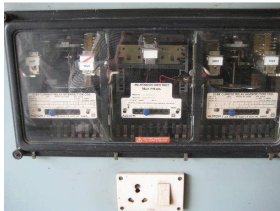
6020 Figure 6.2 Protective relay
