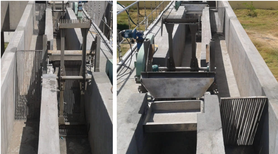
Figure 3.12 UNIDO type arc screen
