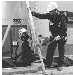
Figure 9.8 Photo showing typical confined space entry
