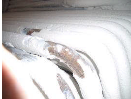
5155 Figure 5.4 Silicon dioxide deposits on boiler tubes
