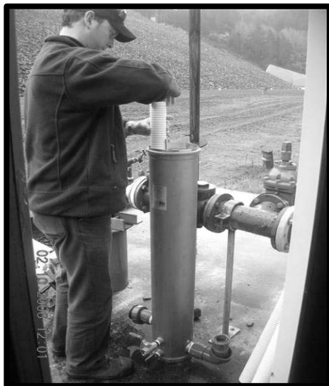
Figure 9a: Cartridge filter system
