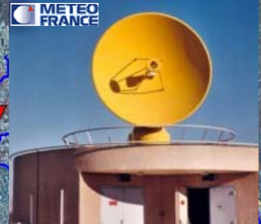
Rain monitoring by radar
