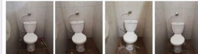
Bathroom B During installation
