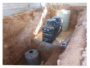
tank for a basic treatment. Waters are then processed in a second tank by infiltration between the various layers of the media Biorock. This medium is specifically considered to endeavor purifying local bacteria's fixation. Cleaned wastewaters are then reused to drip-water a hundred-tree orchard.
