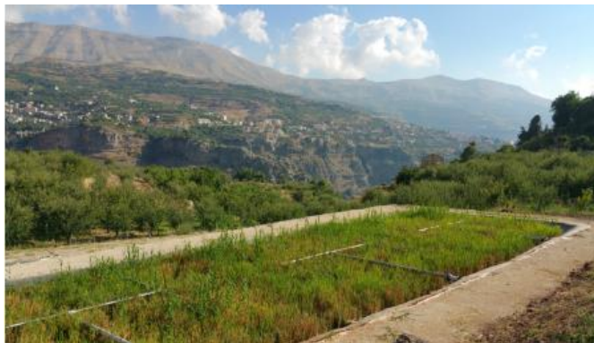
Constructed wetland, Bcharré
