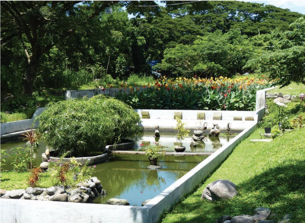
*Figure 17. This natural disinfection pond at Dumaguete City's sewage treatment facility serves as an indicator pond where fish are used to demonstrate the purity of the water.*
