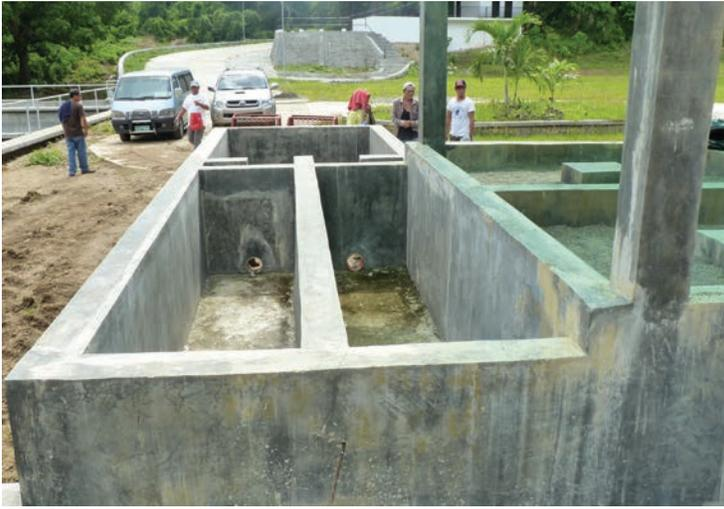
Figure 7. Grit chamber at the San Fernando, La Union septage treatment facility.
