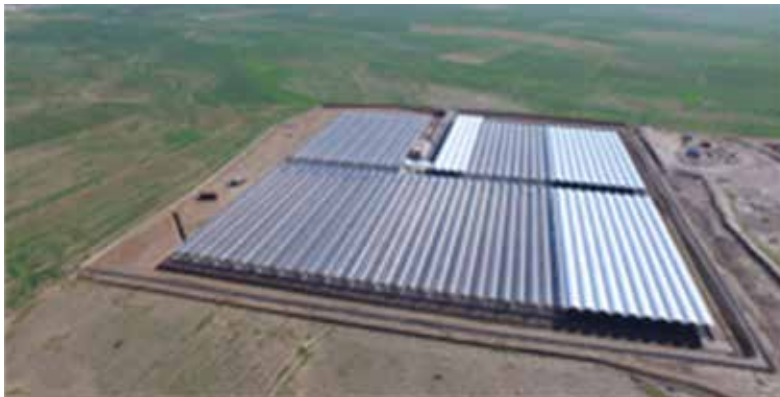
IMAGE 1.1 Solar sludge drying station. SOURCE: RADEEMA.
