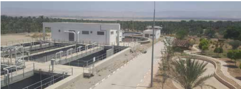
IMAGE 5.2 Jericho WWTP and surrounding date palm farms. Photo: I Abu Seiba
