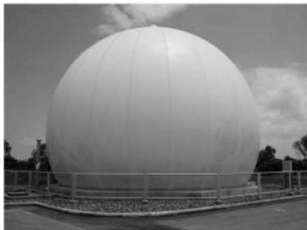
Figure 4.18 Biogas storage tank made of polyethylene, Rayong Municipality, Thailand ( www.cogen3.net )
