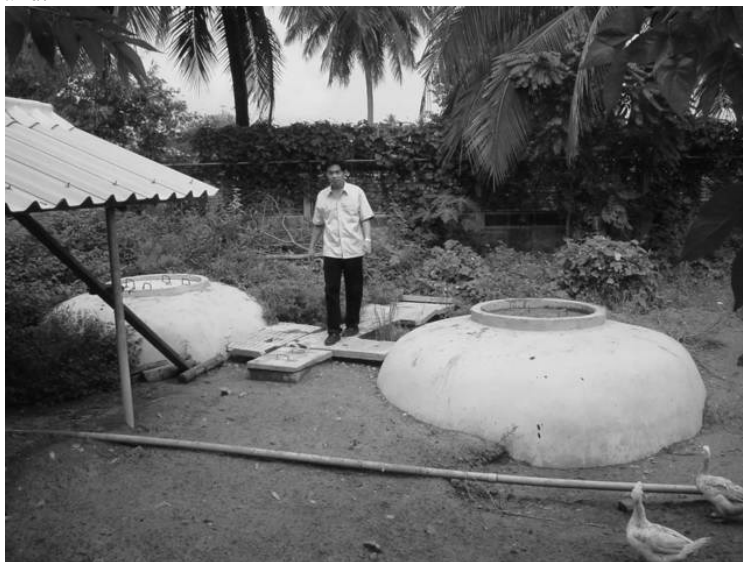
Figure 4.6 Fixed-dome digesters treating piggery wastewater, central Thailand
