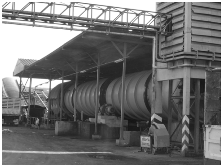
Figure 3.18 A DANO composting plant in Bangkok
