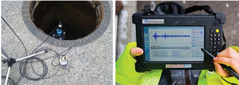
Figure 8.1 Trunk main correlator components and software. (Source: Gutermann)
