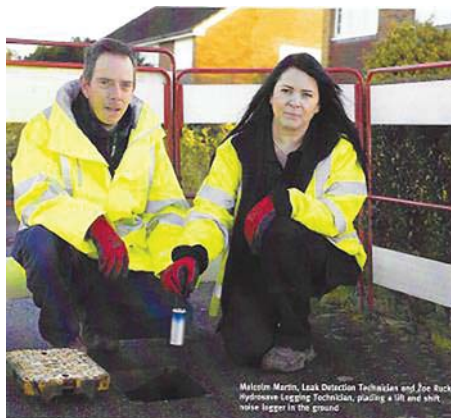
Figure 17.13.2 Deploying a noise logger. (Source: Gutermann)
