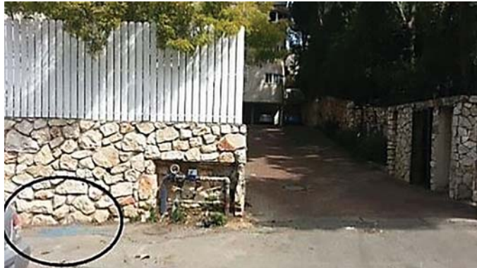
Figure 17.12.7 Leak position marked in blue by contractor. (Source: Gutermann)
