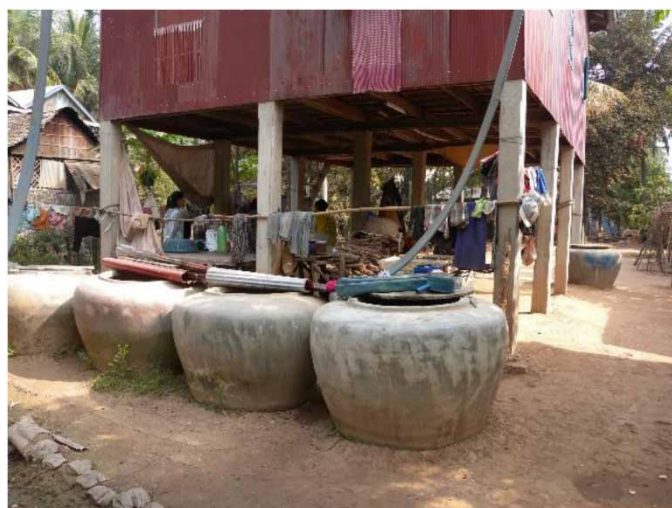
Figure 2 | Traditional rain water tank (Pieng in Khmer).
