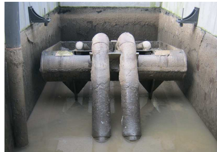
Self-priming siphon for the first stage
