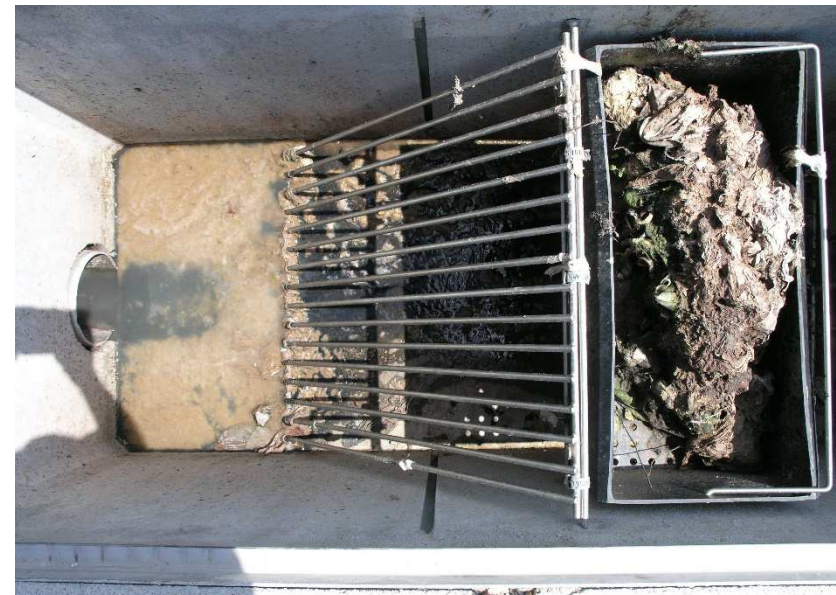
Manual system with a slanted screen made of stainless steel.
