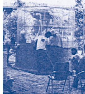
Partially rendered tank
