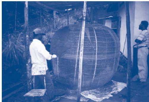
Partially rendered tank
