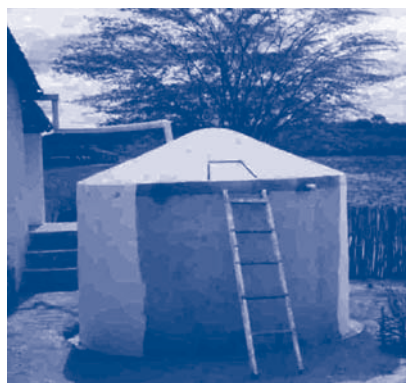
Finished tank being painted
