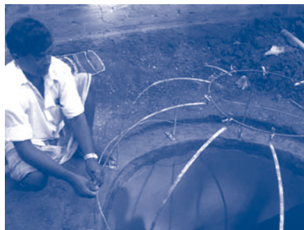
Fixing the frame for the dome
