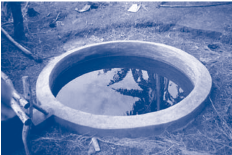
Underground tank with sloped ring beam
