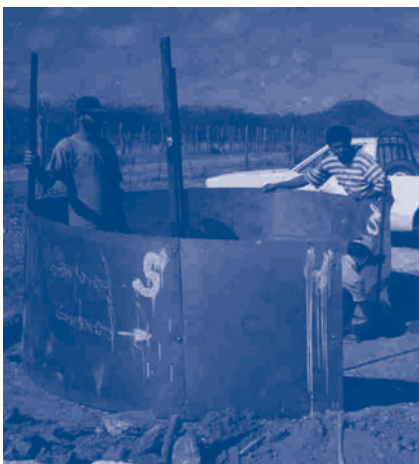
Screwing together the steel sheet form
