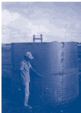
Steel sheet form, wrapped by wire mesh and galvanised wire
