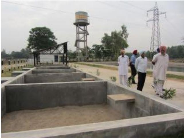
**Figure 4-2** Sludge drying beds, with the third oxidation pond in the background.
