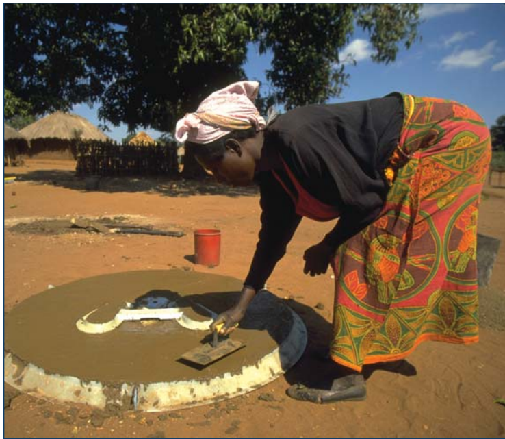
Making a cement slab for a latrine, Zambia ©UNICEF/HQ98-0928/G. Pirozzi
