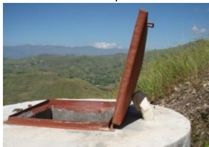
Photo 30: Pierre supportant la porte
