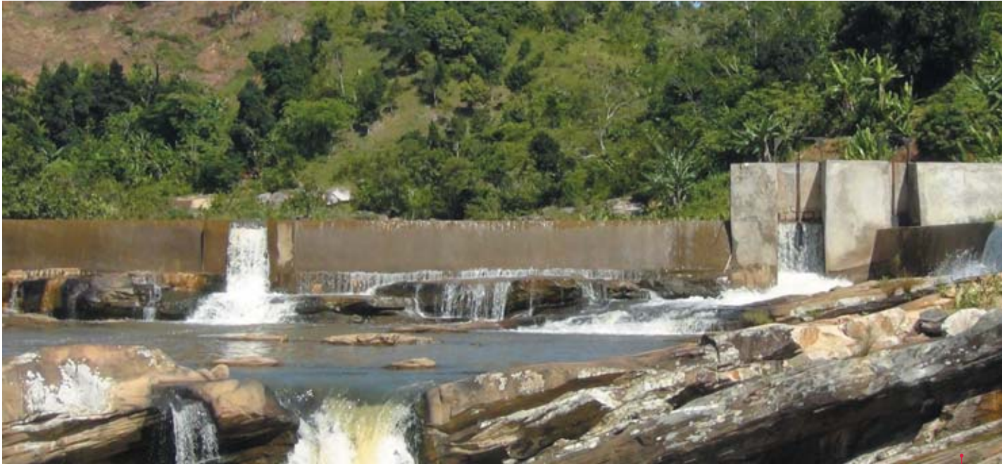
Sahasinaka hydroelectric dam - Source: GRET
