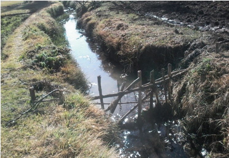
Figure 7: Traditional way of raising water levels in canals at Dessie-Zuria scheme.
