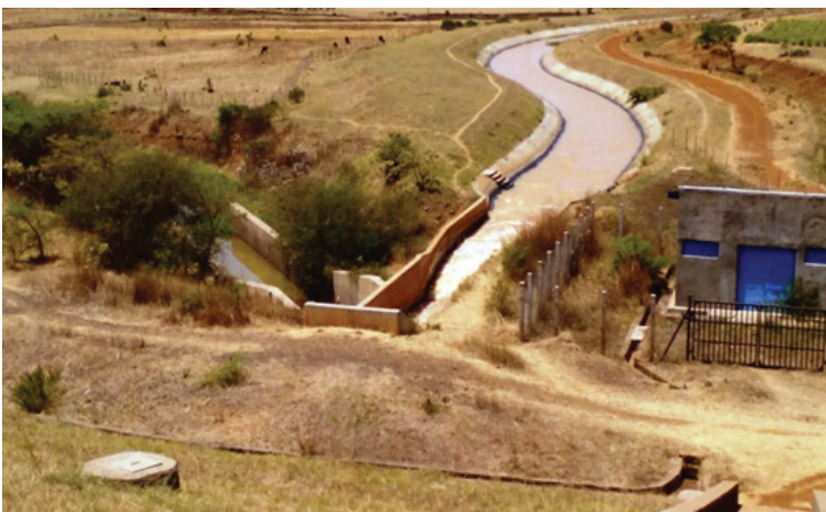
Figure 8: Koga scheme dam outlet and off taking main canal.
