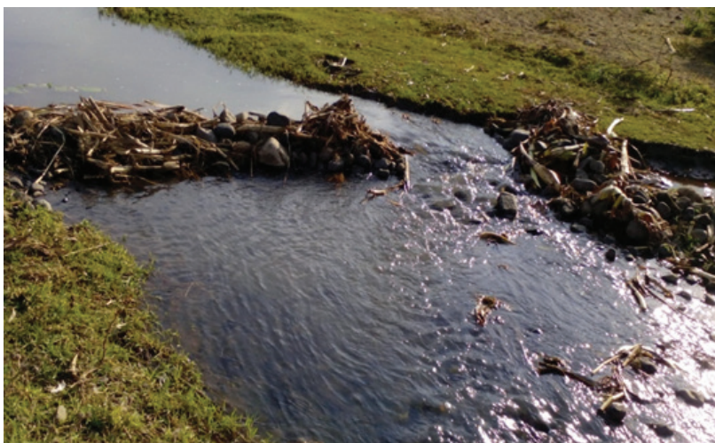
Figure 6: Traditional flow control with debris and stones at Waro scheme.
