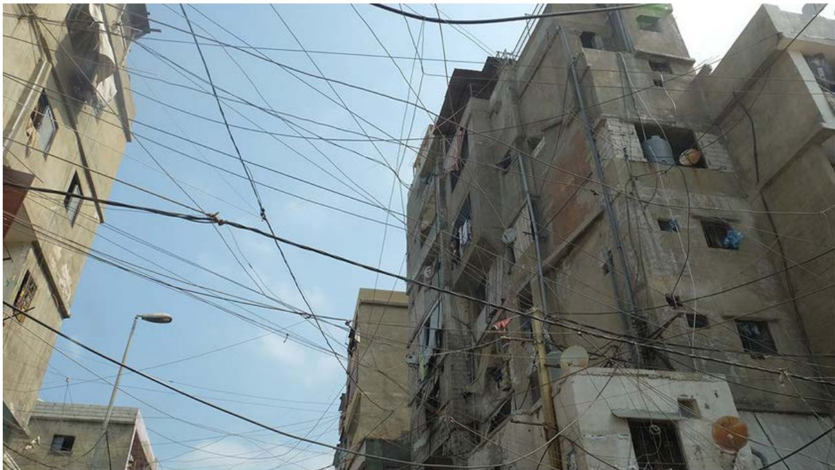
Illegal electricity connections are common in Beirut
