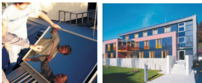
Figure 5 • Glazed flat plate collectors
