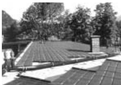
Figure 4 • Flat plastic plate collectors for swimming pool water heating
