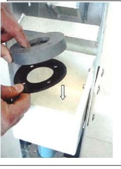
4) Place seal and flange into the water tank.
