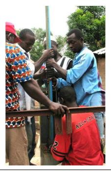
3) Raise the first section of the riser pipe.4) The double socket of the second section of the riser pipe should be at the level of people's shoulders
