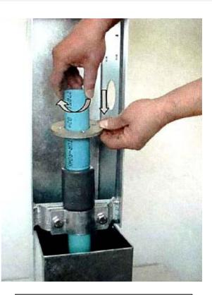
2) Screw connecting pipe for water oulet on last riser pipe unit
