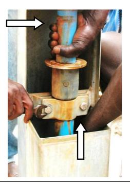
1) Dismantling the riser pipe is made with the help of the steelclamp fixed at the bottom of the pump body
