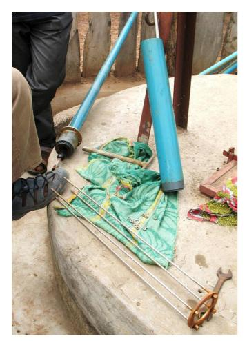
1) Once all cylinder components have been checked and cleaned, reassemble them
