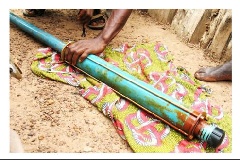
1) Once the last riser pipe section and rod is dismantled. Lay down the cylinder of the pump unit. Keep it away from sand and dust.
