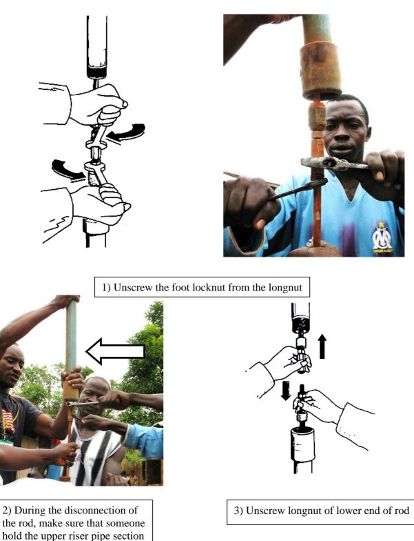
Proceed the same way to disconnect all the riser pipe sections and rods.
