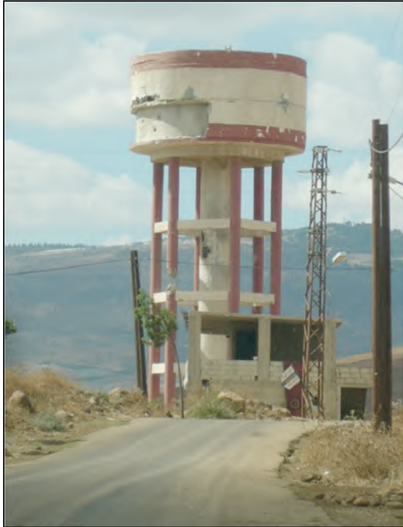
Figure 5.3 Wazzani Booster Station Reservoir suffering direct (and deliberate) damage, 2006 (SLWE 2006).
