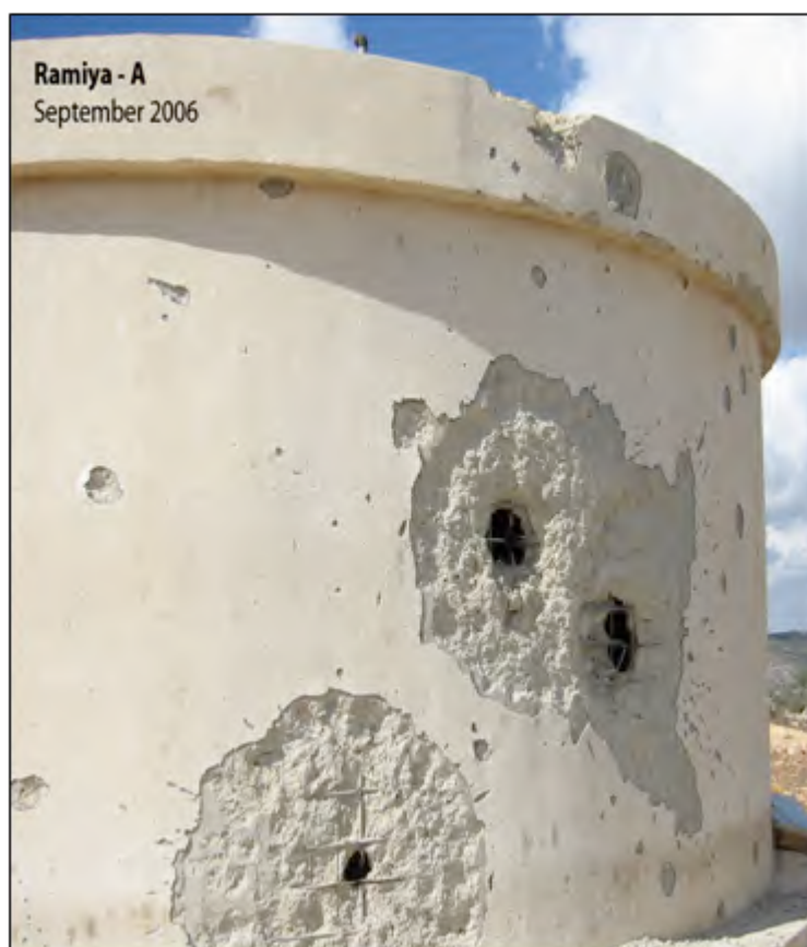
Figure 5.2 Water reservoirs in Lebanon damaged during the 2006 Summer War, showing a range of the nature of the damages. Siddiquine: no direct damage to reservoir; Chama'a: 'indiscriminate' and 'deliberate'; Ramiya: 'deliberate'. (All photos by authors. See also Annex D).
