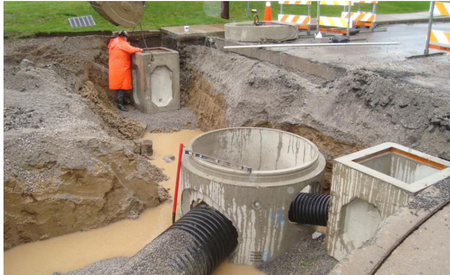
Figure 5: Connection within manhole.
