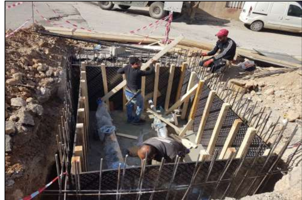
Constructing a manhole in Labweh
