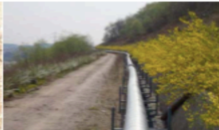
Landfill gas transport pipe being installed on slopes
