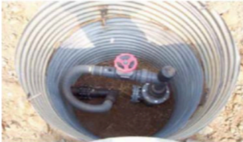
Landfill gas extraction well installation
