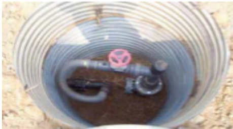
Landfill gas extraction well installation
