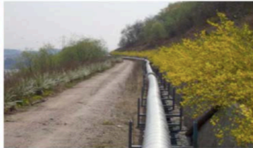
Landfill gas transport pipe being installed on slopes
