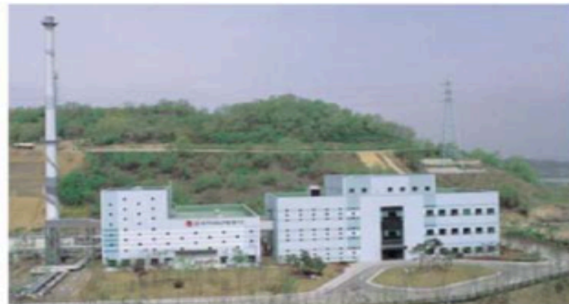
Heat production facility using landfill gas
