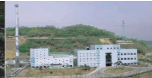
Heat production facility using landfill gas
