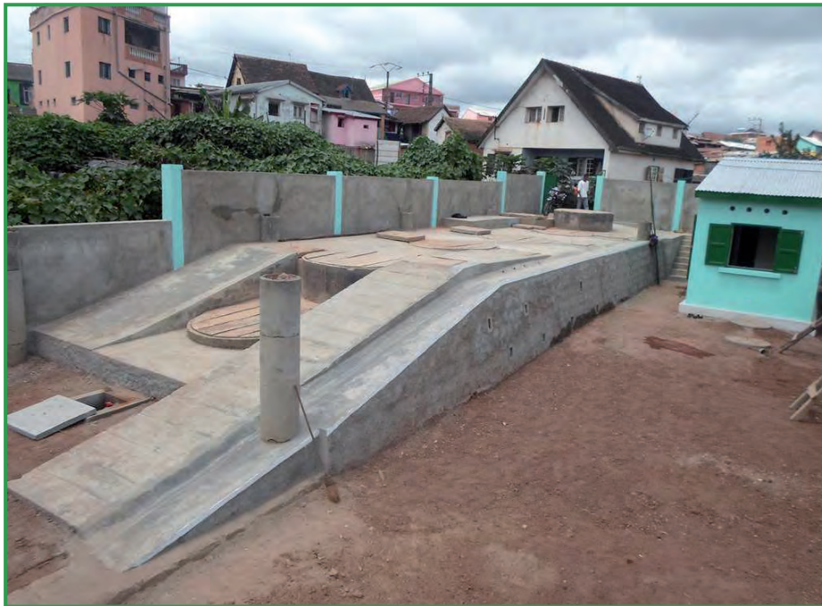
Figure 9 - Station de traitement de Tanjombato
