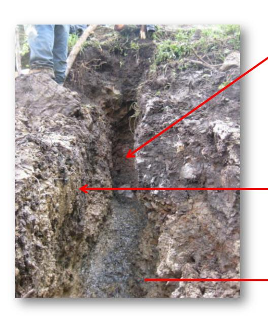
If possible, continue digging away from the spring until water is no longer seeping in from the end of the trench here
