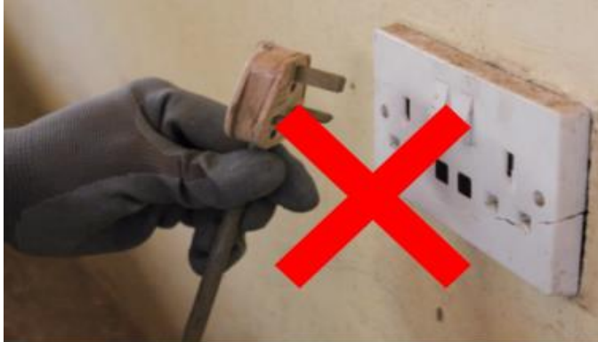
Figure 11: No re-use screening via plug-in and function test
