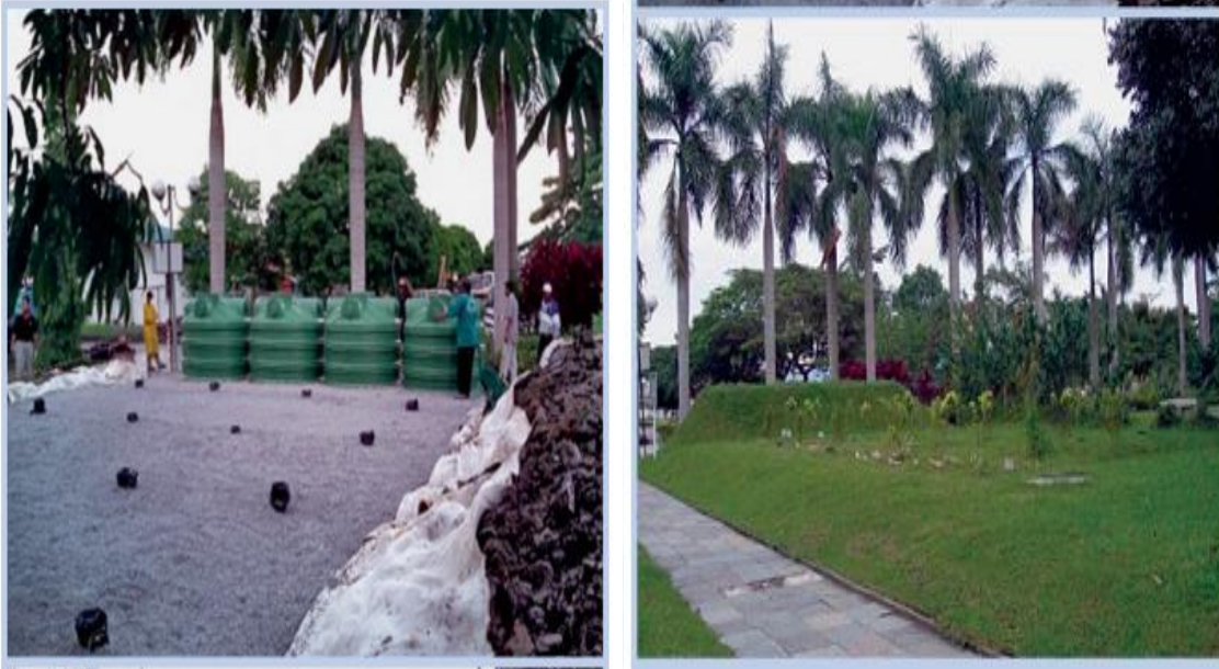
3-12 Aerobic filters and planted filter under construction and completed
