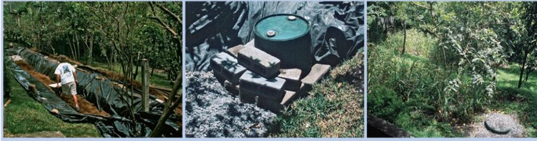
3-7b Build up of 1st Reed bed
