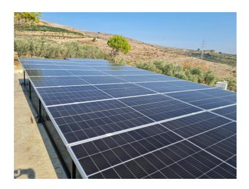
Equipping the Water Station of Al Blat- Meryata with a Solar pumping System to operate a 17.5 HP submersible pump
