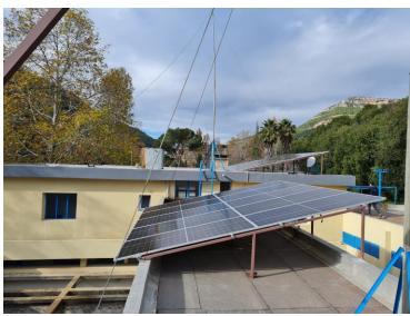
Equipping the Water Station of Kferhalda- Batroun with an Off- Grid Solar System, providing 50 KVA during the Day and 25 KVA at Night shift
