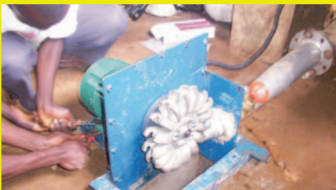
Installation of the turbine (Kathamba).
