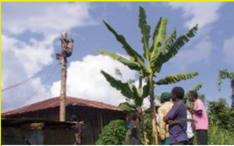
Installation of electric posts in Kathamba.
