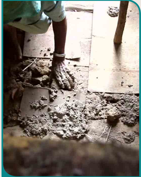
Fly-proofing the latrine floor
