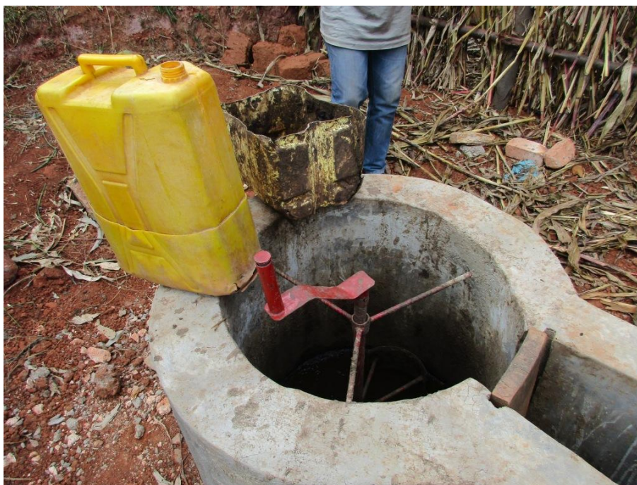
Figure 19 – Biodigester inlet, jerrican and basin – or ‘cut jerrican’ (ENEA consulting)
