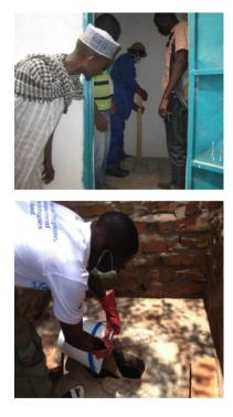
**Figure 9 and 10.** Measuring the height of faecal sludge (left) and pouring additive in a pit (right) during field trials in Chad. (Source: Christophe Grange, UNHCR)
