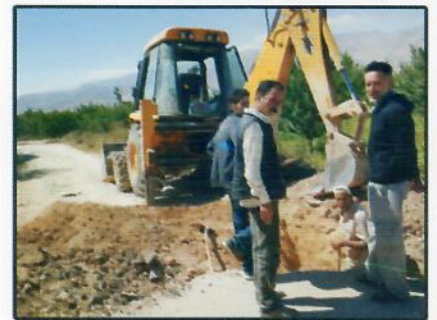
Rehabilitation of Bejjeje-Jabboule Network
