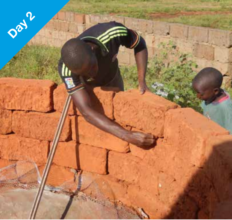
Above: construct the mould with clay blocks in + 9 rows to reach a height of 1.70 m. Below: apply 1 layer of clean wet sand for a smooth inside surface of the mould. Use a spirit level to make a vertical wall.
