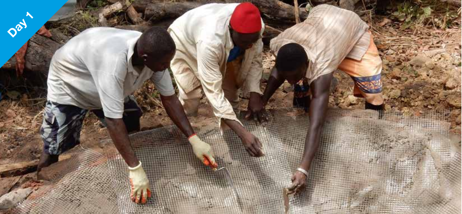
Cut and adjust the chicken mesh on the first layer of the wet mortar and cover it with the second layer of mortar (2nd bag). The chicken mesh serves the purpose of reinforcement inside the cement.
