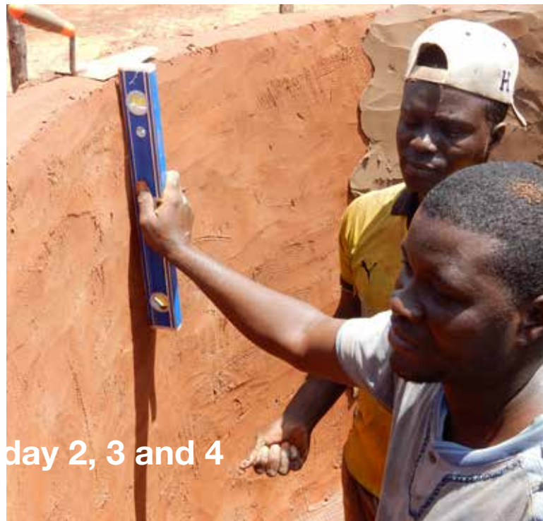
Above: construct the mould with clay blocks in + 9 rows to reach a height of 1.70 m. Below: apply 1 layer of clean wet sand for a smooth inside surface of the mould. Use a spirit level to make a vertical wall.
