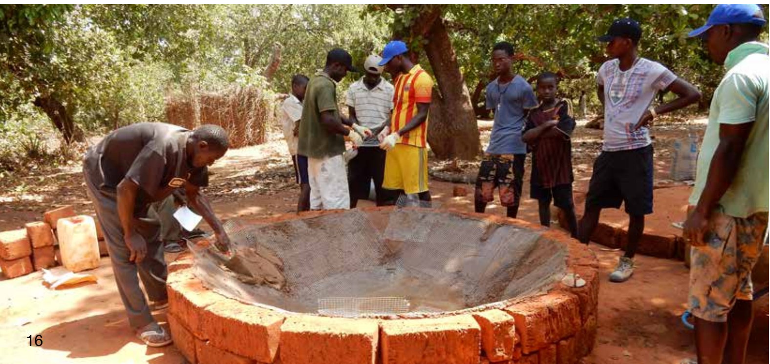
Cut and adjust the chicken mesh on the first layer of the wet mortar and cover it with the second layer of mortar (2nd bag). The chicken mesh serves the purpose of reinforcement inside the cement.
