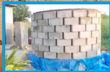
Cement blocks can be used, when clay blocks are not available.
