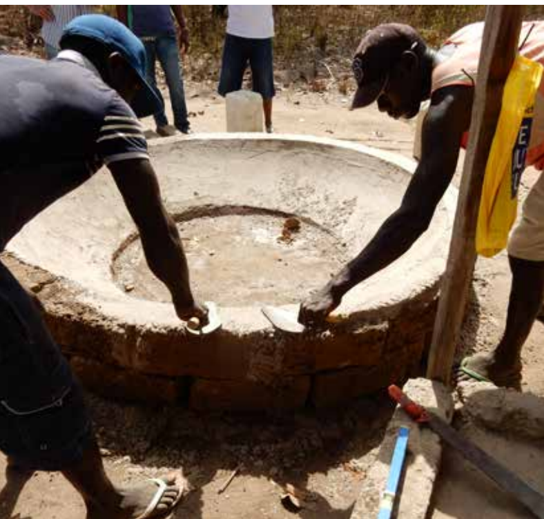
Above: adjust the clay blocks in the upright position.
