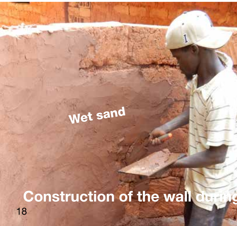
Above: construct the mould with clay blocks in + 9 rows to reach a height of 1.70 m. Below: apply 1 layer of clean wet sand for a smooth inside surface of the mould. Use a spirit level to make a vertical wall.
