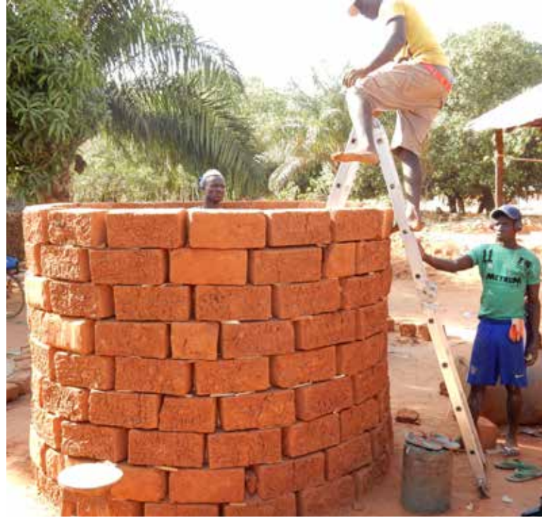
Above: construct the mould with clay blocks in + 9 rows to reach a height of 1.70 m. Below: apply 1 layer of clean wet sand for a smooth inside surface of the mould. Use a spirit level to make a vertical wall.
