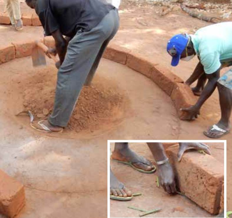
Above: adjust the clay blocks in the upright position.
