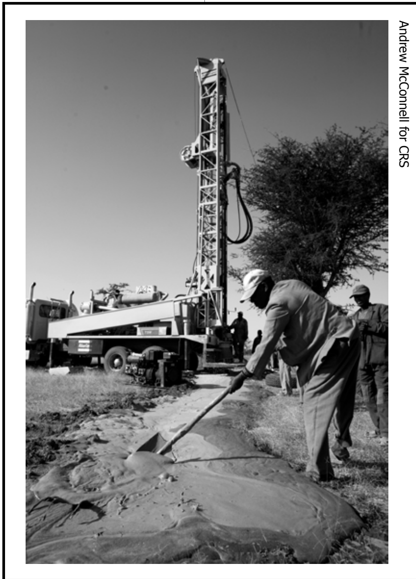
A rotary drilling rig using mud slurry to prevent the well from collapsing in Ethiopia.
