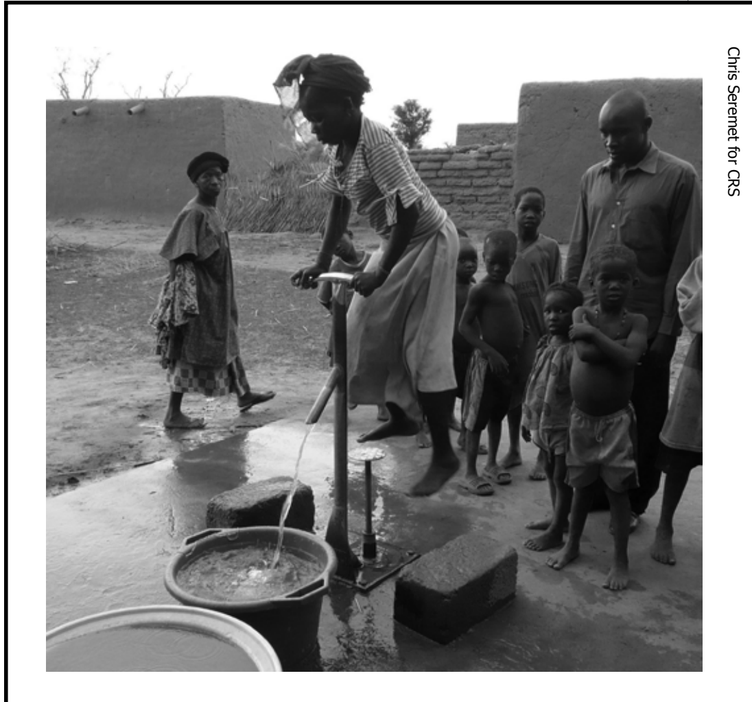
A Vergnet footpump being operated by a woman in Mali.
