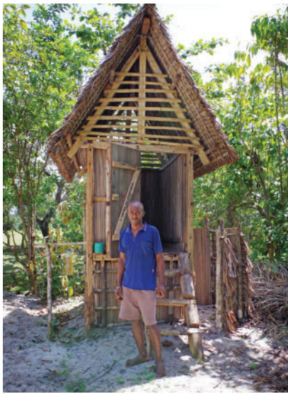
In Ampasinimaningory village, Analanjirofo Region, raised bamboo structures were built in some coastal areas.
