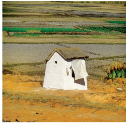
Different designs have been made to deal with high groundwater and vulnerability to flooding. In Vakinankaratra Region (CARITAS Project), there were mud structures with raised latrines in low-lying: the door and floor level is about 70 cm from ground level.
