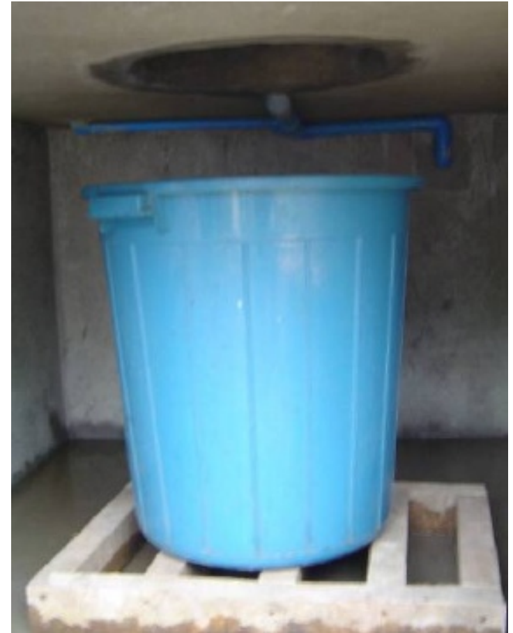
Drums for collection and storage of faeces, Philippines
