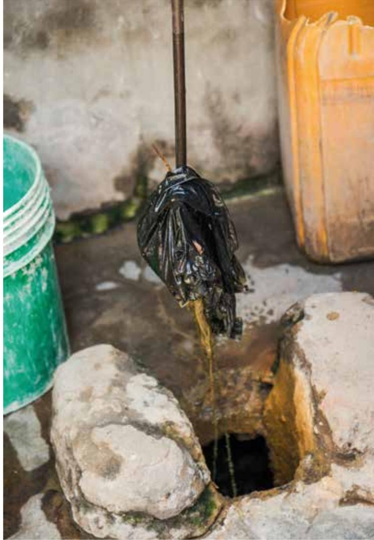
Removing plastic waste before pumping
