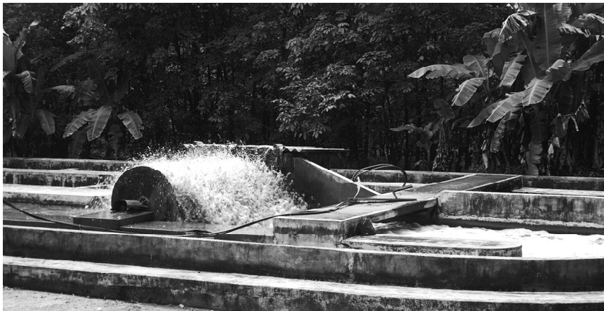
Fig. 53. Oxidation ditch operated at a rubber factory in Kerala / India [photo: Sasse]
