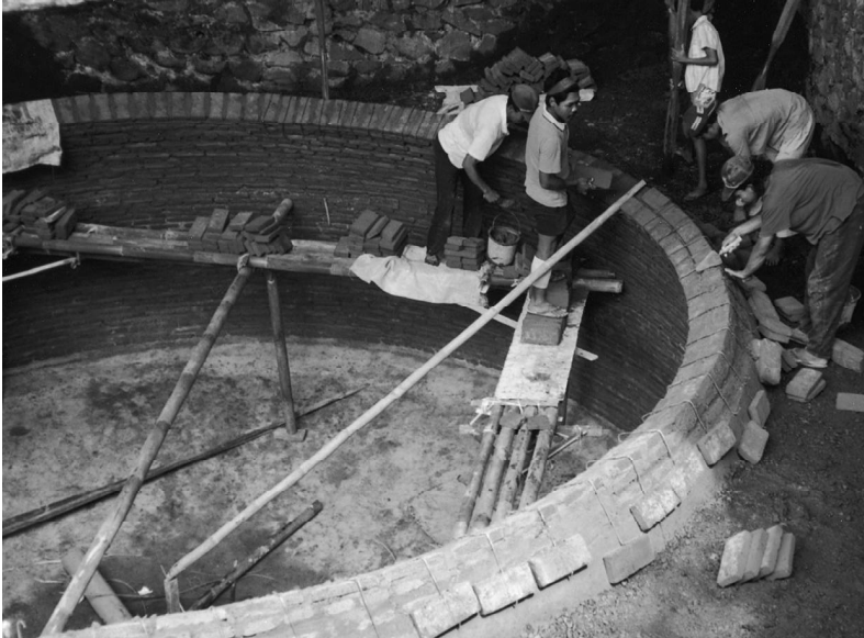
Fig. 58. This plant had been constructed by LPTP and BORDA for cattle dung in a meat factory in Central Java
