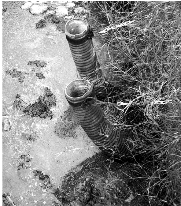
Fig. 54. Flexible pipes for de-sludging. Sludge is discharged by hydraulic pressure when lowering the pipe. [photo: Sasse]
