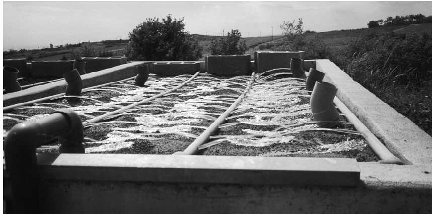
Fig. 38. Vertical filter during charging. Constructed above ground by Nature & Technique, D. Esser, for a cheese dairy in southern France. [photo: Sasse]
