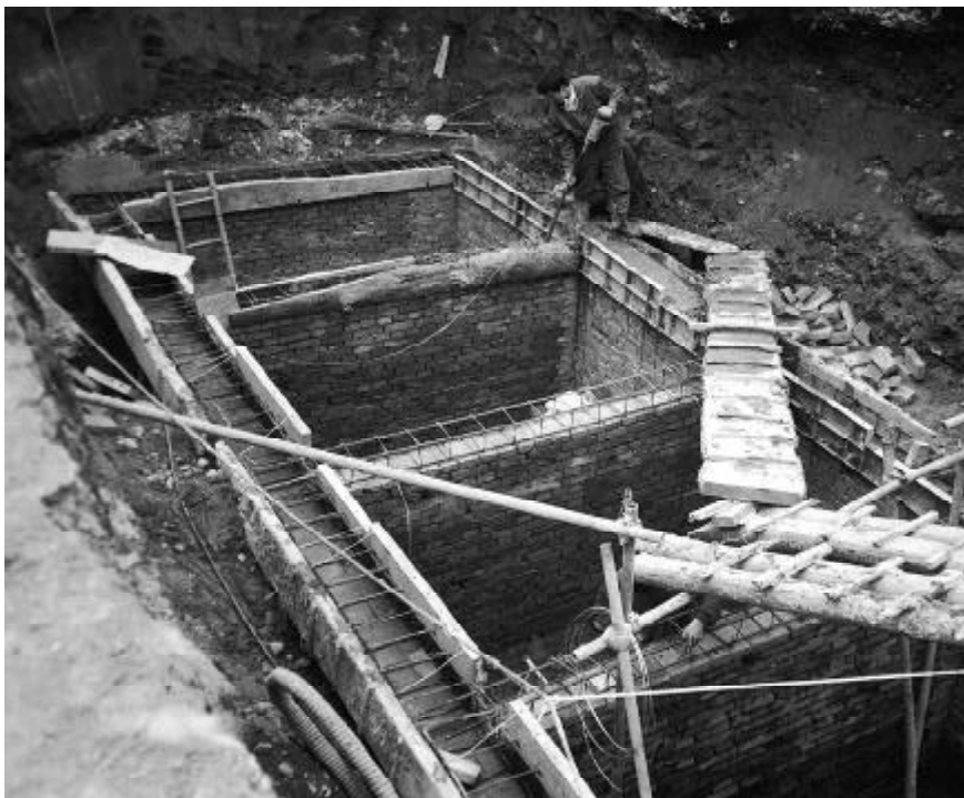
Fig. 3. DEWATS anaerobic filter under construction. Planning and supervision by CEEIC [photo: Sasse]
