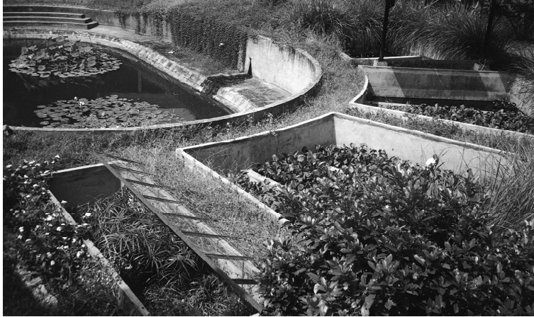
Fig. 48. Wastewater treatment tanks using aquatic plants in Auroville / India. The plant is placed directly beside residential houses. Lizards which live among the water hyacinth take care of mosquito control. The first settling tank is sealed against bad odour by a thick layer of scum on which papyrus grows (see Fig. 46). [photo: Sasse]
